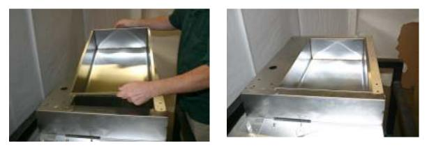
2. Place the blower unit in the well making sure to slide it flush against the wall of the well.
