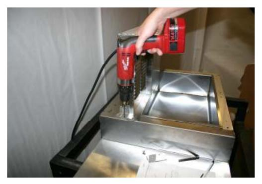
5. Insert and tighten screws provided (SCR008).
