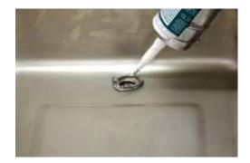
8. Press Drain Cover onto sealant firmly. Then clean any excess sealant from around the Drain Cover. Allow sufficient time to cure (at least 12 hours).
